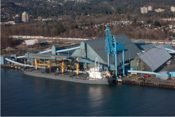
Martin designed and installed five new conveyors at the Vancouver Wharves Kinder Morgan terminal, ranging from 105 feet (~32 meters) to 709 feet (216 meters) in length.
