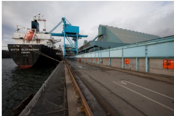
All mineral concentrate storage and handling facilities are fully enclosed to ensure no concentrate escapes or migrates into the ocean.
