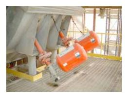
The Martin® Air Cannons installation included Martin® Thermo Safety Shields to protect maintenance workers from exposure to high temperatures.
