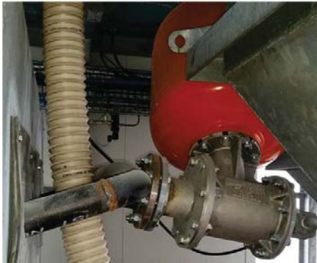
The positive-firing valve requires an air pulse signal from the solenoid to trigger discharge.
