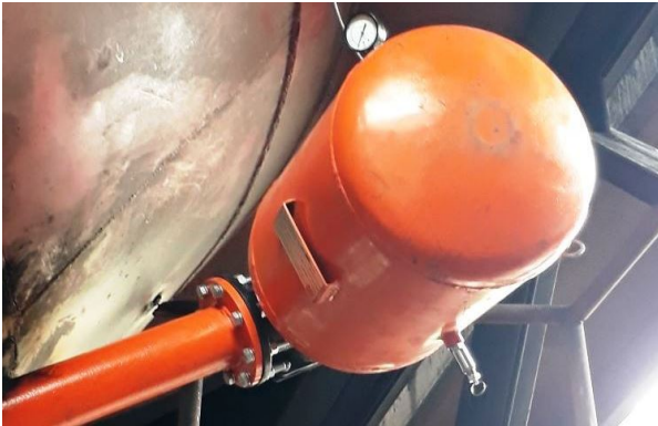
The Martin® BB4 / Master Blaster Air Cannon attaches to a straight pipe assembly extending into the vessel.
