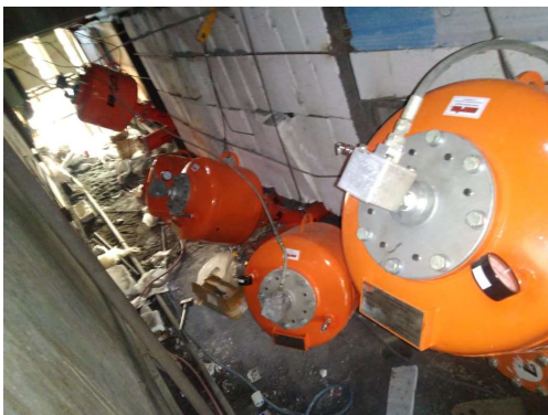
The old nozzles below had to be cut out, while the new orange ones simply slide out from the Y assembly.
