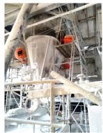
Strategically positioned at critical points around the bin, the four Typhoon Air Cannons prevent accumulation.
