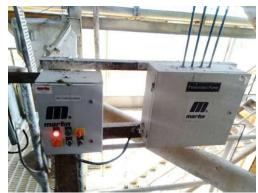
The air cannons can be programmed to fire automatically at specific intervals or manually activated.
