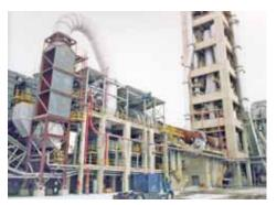
Material buildups in the pre-heater tower at the Holcim Devils Slide Plant led to the installation of Martin® Air Cannons.
