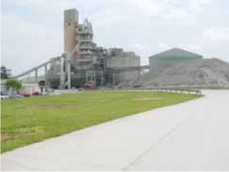
*The CEMEX plant in Knoxville, Tennessee lists capacity of 2,500 tons per day for an annual output of 800,000 tons per year.*
