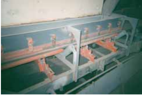
Martin® ApronSeal™ Single Skirting and Martin® Support Cradles were installed.
