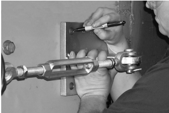
12. Extend spring link assembly to final position and mark holes while pressing blades against belt.
