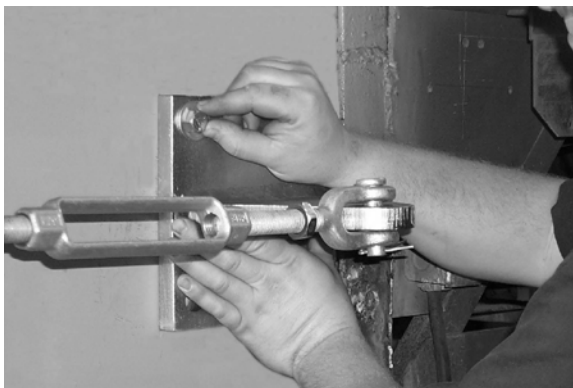
14. Secure top mount weldment to chute wall.
