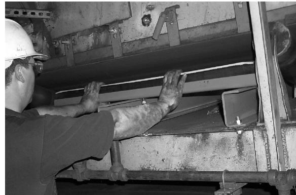
11. Line bolts up with slots and repeat for remaining cross sections. Tighten bolts.
