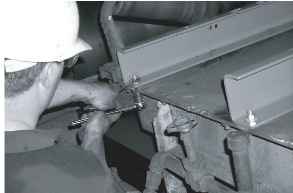
7. Measure between cross support channels. Make sure the cross-support is square.
