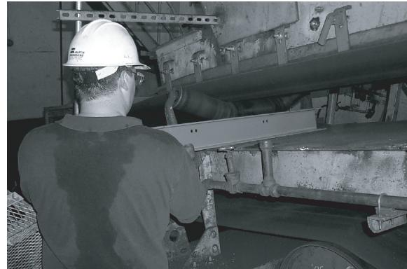
1. Slide cross-supports under belt in pre-determined location and align with marks.
