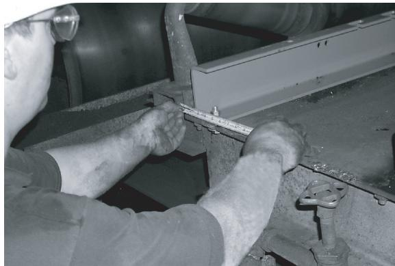
6. Measure the distance from the idler to the first cross member bolt. Verify the dimensions and tighten the bolt into place. (Refer to Figure 3 for Martin® Impact Cradle LD dimensions and Figure 4 for Martin® Impact Cradle MD dimensions.)
