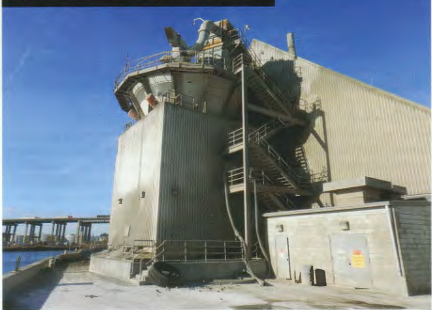
Barges dock several times a week to drop off raw materials
