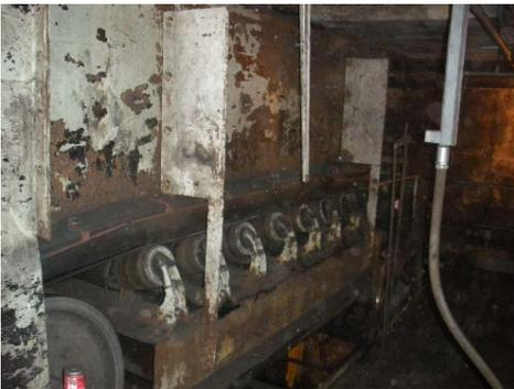
*The poor condition of the chutes loading the plant's belt feeders led to a significant coal spillage problem.*
