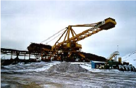
Carryback created problems for the reclaim conveyor in the QCM Shiploading Facility.
