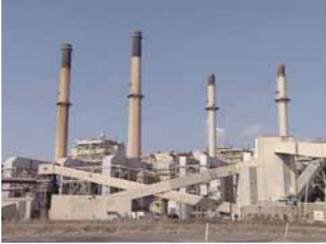
The AmerenUE Meramec plant is a four-unit, 865MW facility fired with PRB coal.
