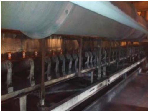
The solution has proven very effective, dramatically reducing dust, carryback and spillage.
