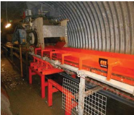
Martin recommended a complete upgrade of the transfer points.
