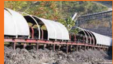
Covers left off after maintenance can expose workers to hazards.
