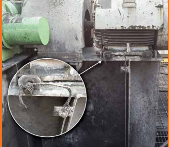
This electric drive motor is poorly bonded to the metal structure, and so poses a hazard if the conveyor was struck by lightning.
