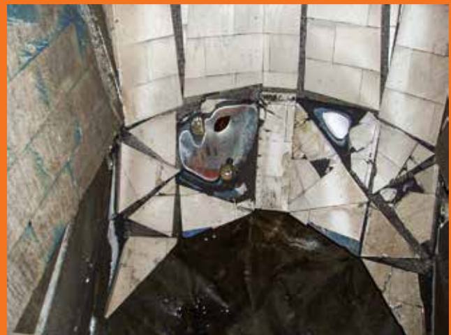
Loading spoon chute liner damaged from direct material impact.
