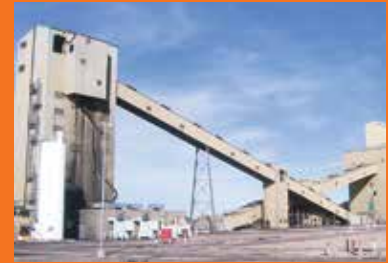
Typical conveyor gallery, exterior view.
