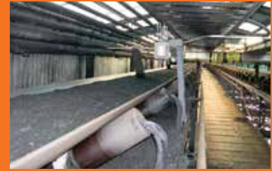
Typical conveyor gallery, interior view.
