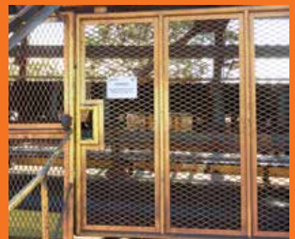
A gate to a conveyor walkway is controlled with an RFID sensor.
