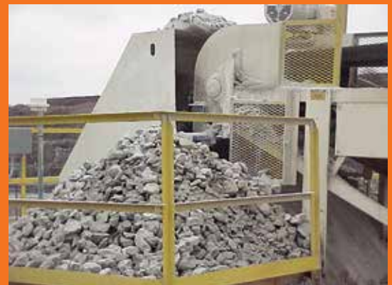
A disabled plugged chute detector results in the accumulation of materials on the walkway and the increased risk of worker accidents.
