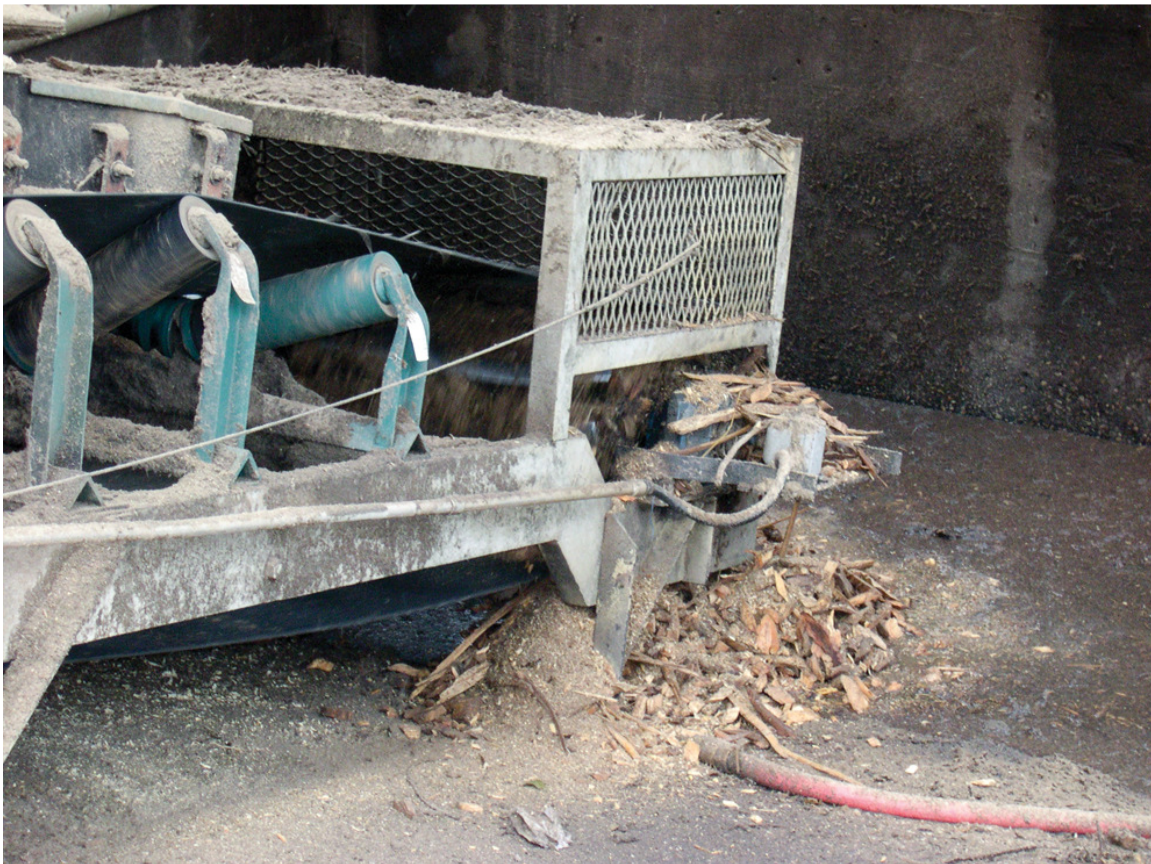
Figure 1.1 Tail Pulley Suffering From Entrapment.
