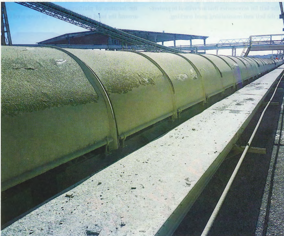
5 This cable tray blocks access for efficiently replacing idlers
