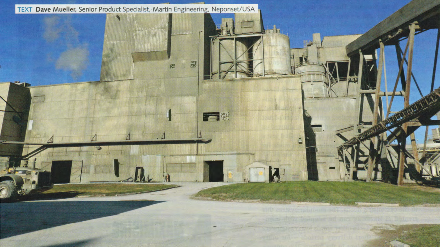
1 Conveyors transporting bulk materials have different entry points into the plant
