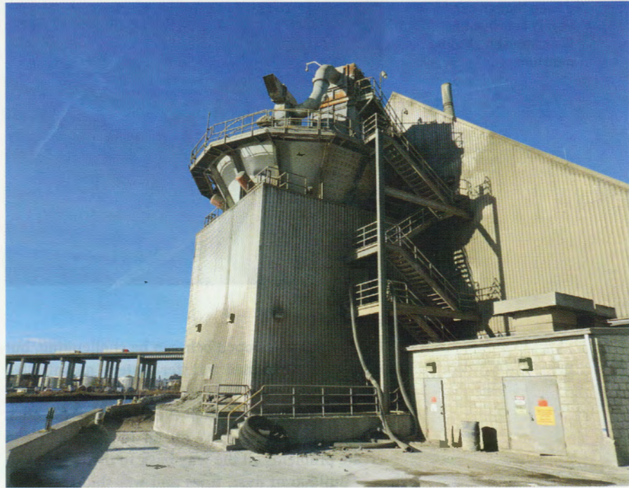
2 River barges dock several times a day to drop off raw materials
