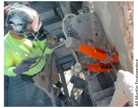
A technician makes the final tensioning adjustment this CleanScrape™ blade will need for the life of the cleaner
