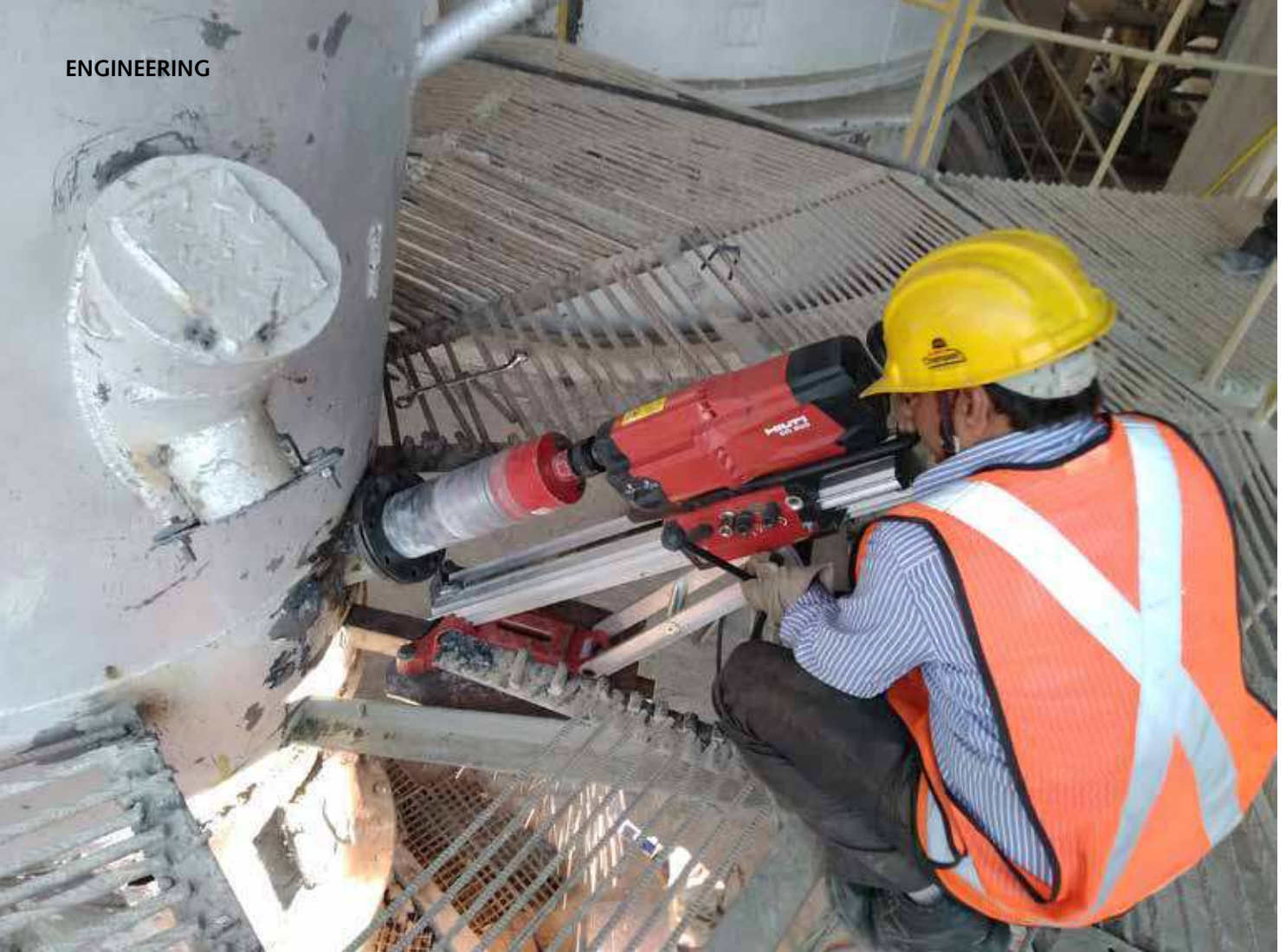
2 Core drilling during production by a trained technician
