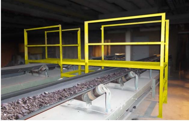
Figure 4. A designated crossover designed for that purpose is the only safe path to the other side.
