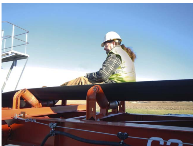
Figure 2. Riding a conveyor is hazardous, even in locations where man-riding is an accepted practice.
