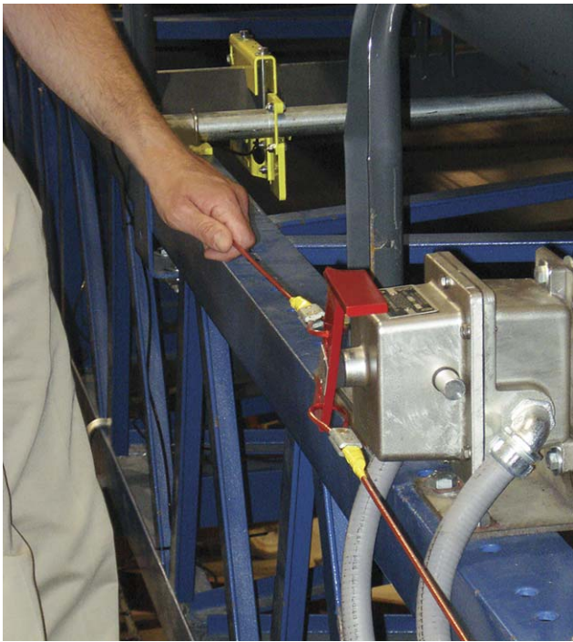
Figure 5. Safety equipment such as pull stops and emergency switches are vital to conveyor safety.
