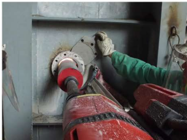
Core drilling during production by a trained technician.
