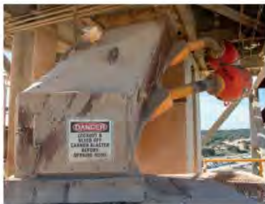
Figure 6. Air cannons prevent clogging and help direct the flow of material.
