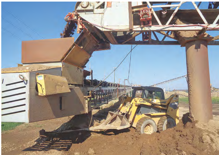
Figure 6. Raising belt speeds and volumes have consequences for transfer chutes and cleanup.
