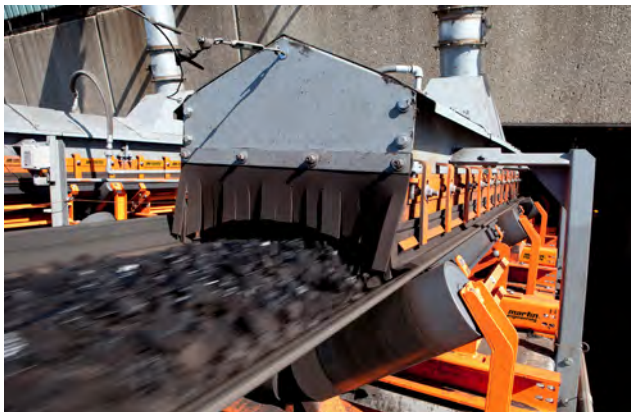
Figure 1. Adjustments in belt speed and load volume should be accompanied by an in-depth assessment of the system.
