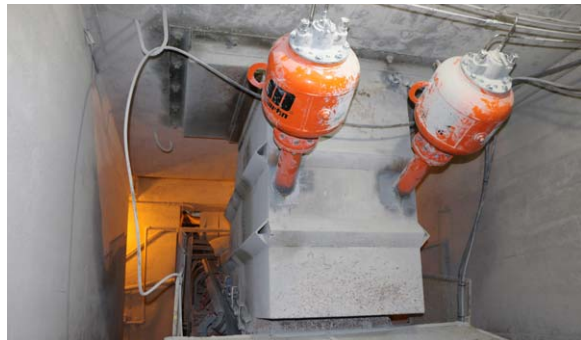
One cannon was located at the head of the conveyor, with two others at the tail.
