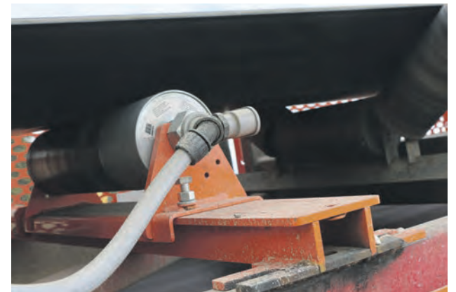
The Roll Gen system uses energy from the moving conveyor belt to generate power for lighting at night.
