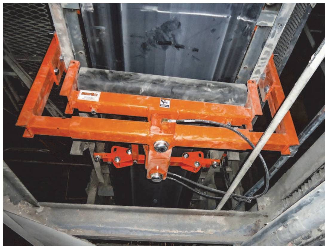
Each conveyor was fitted with a Martin® Tracker™ for the return side, to help reduce edge damage, prevent spillage and extend belt life.
