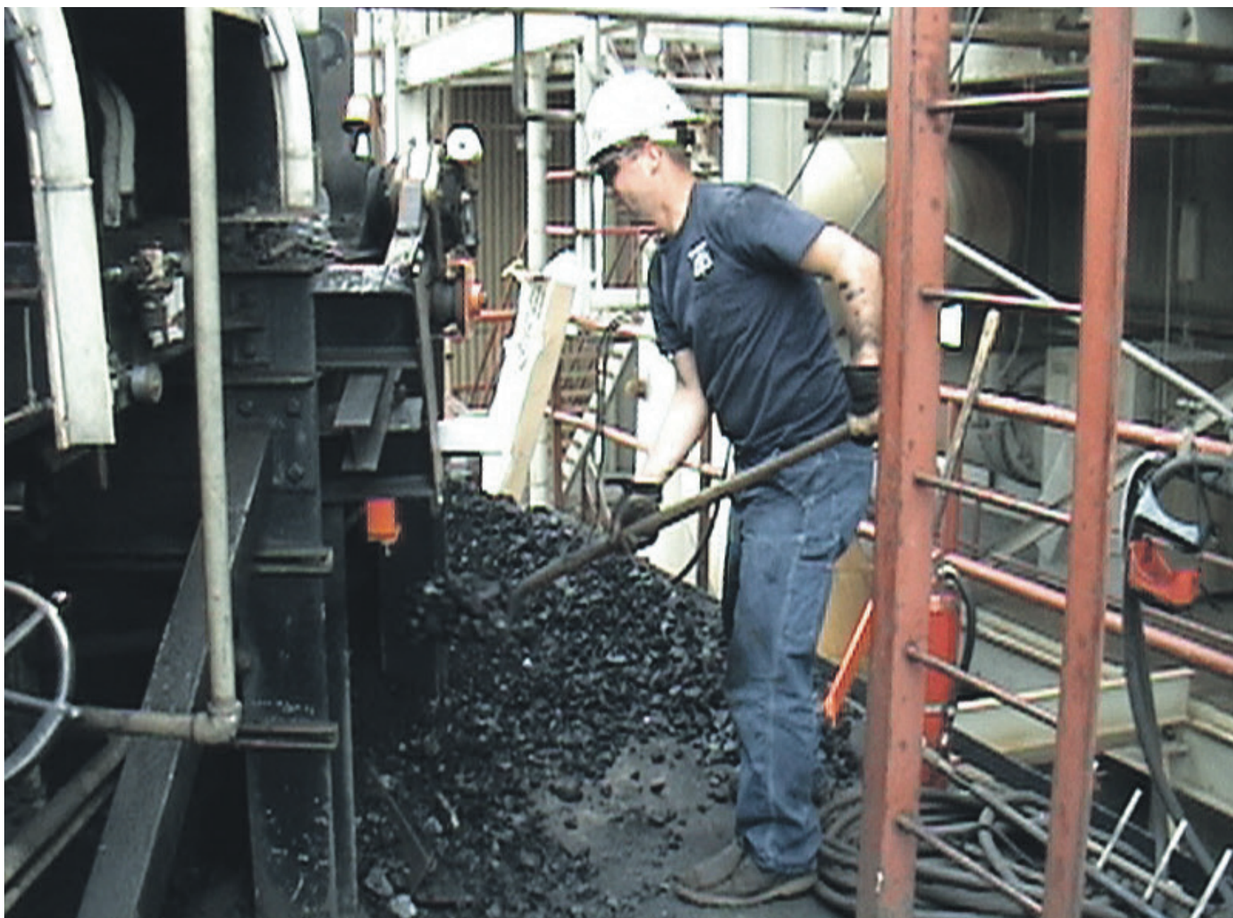
Cleaning up spillage exposes workers to a potential hazard area from the moving conveyor.
