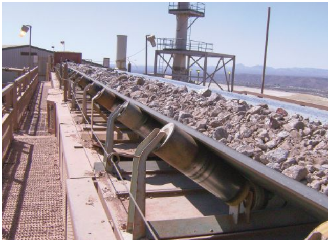
A belt conveyor is a large, complex and powerful system.
