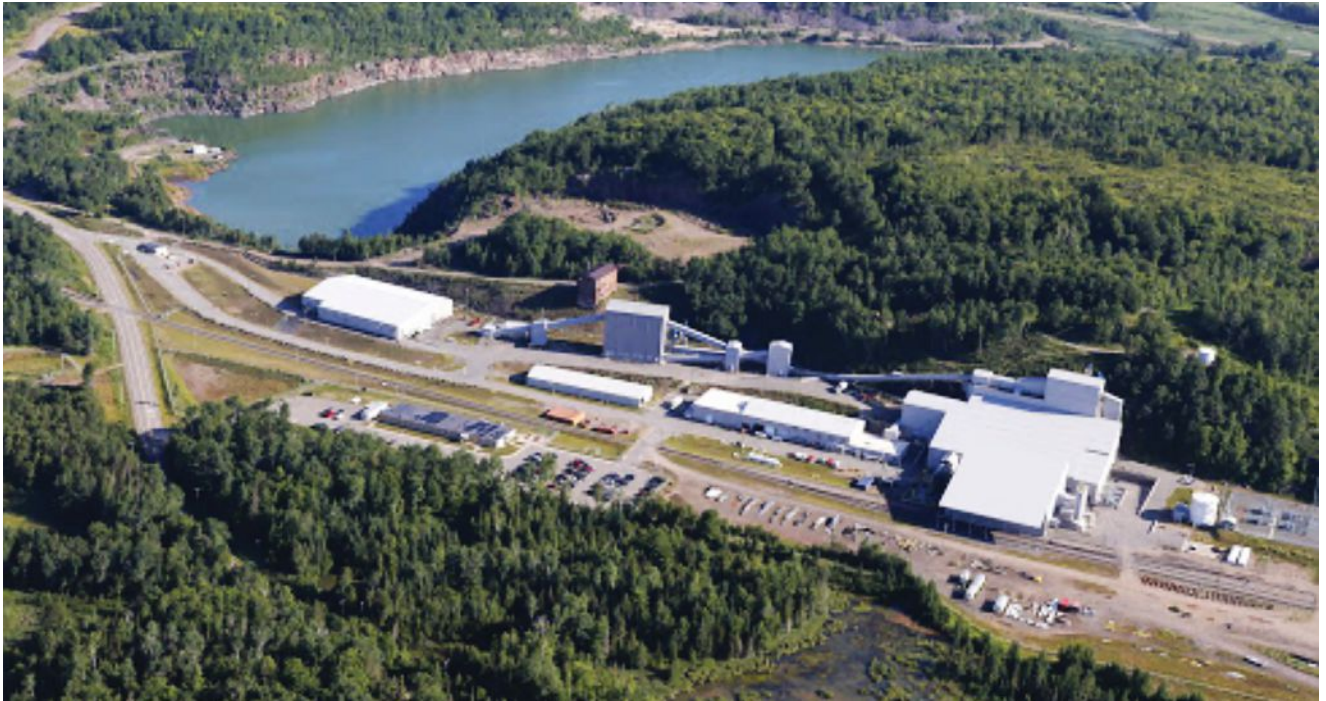
Located on the sight of an old ore processing mill, Humboldt Mill was retrofitted with the latest technology.
