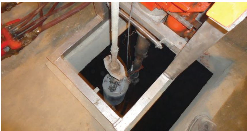
The cleaning crew set up the whips outside of the access hatches.
