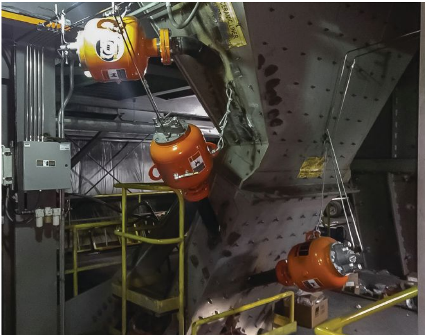
Strategically positioned at a 30° angle, the cannons keep material flowing.
