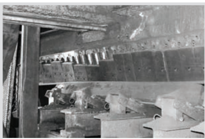
Sectional skirting can wear unevenly, causing gaps and increased maintenance.
