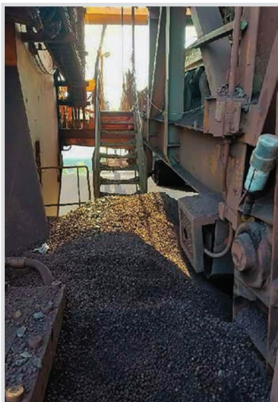
Cluttered stairs and walkways created a workplace hazard.
