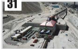
ABB completes commissioning of the world's most powerful conveyor system
