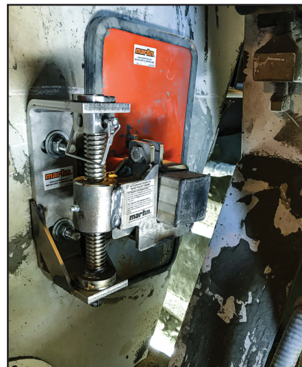
The CS2 typically requires just one re-tensioning during its lifespan, helping to reduce cost of ownership.
