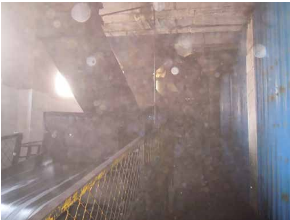
Access to the #111 transfer point was seriously limited by the lack of visibility caused by dust.
