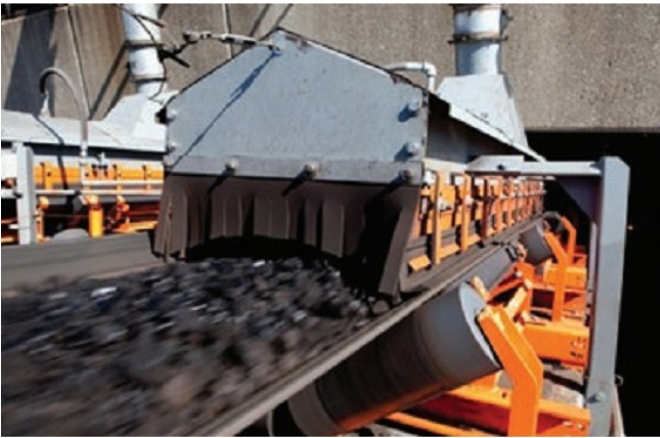
Copyright: Martin Engineering A properly configured conveyor minimizes emissions for improved safety and easier maintenance.
