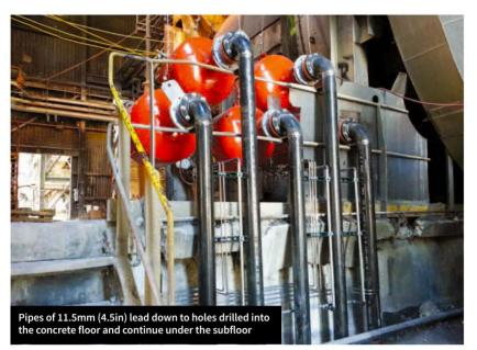
Lehigh Hanson's first solution had five cannons with standard OEM piping leading directly to problem areas on what operators dubbed the 'hot wall', which was located right next to the hottest part of the cooler. The area has an average sustained temperature of 65-74 °C (150-165 °F), which makes maintenance during operation impossible. Even during short downtime events for emergency repairs, high-heat personal protection suits were still required.
