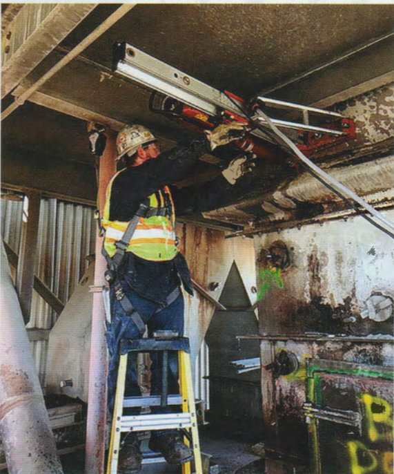
New technology allows air cannons to be installed and serviced without a process shutdown.
