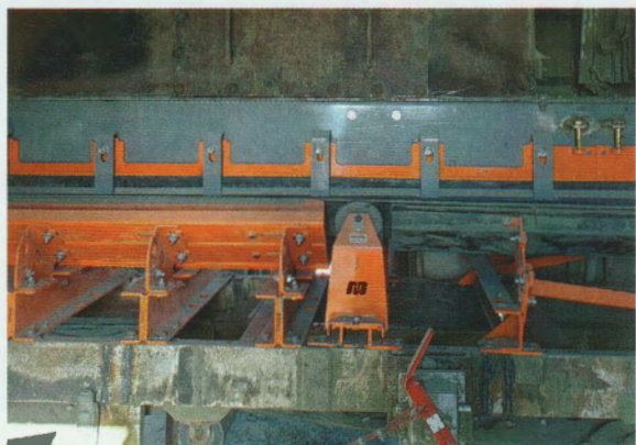
Integrated modular components work
