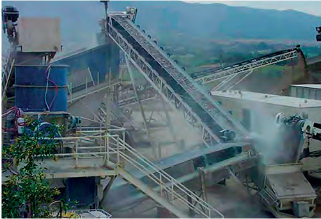
Figure 1. Dust control for operations with several conveyor transfers can be a serious challenge.
