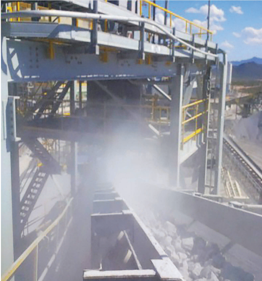
Raw bulk material drops onto a moving conveyor belt, creating dust and spillage.
