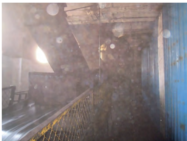
Figure 5. Access to the #111 transfer point was seriously limited by the lack of visibility caused by dust.
