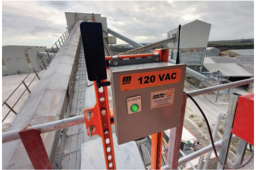
The cellular gateway receives data from up to 200 N2 PI's and sends it to a cloud-based server.
