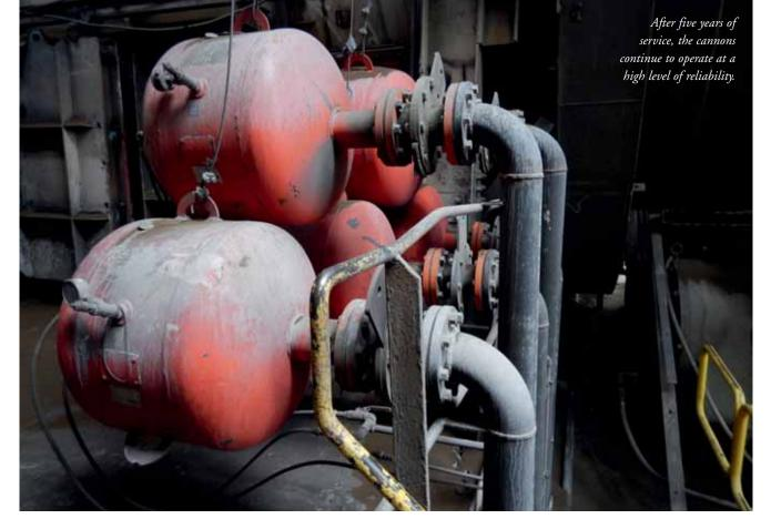
has to travel further, we installed the powerful 150-litre Hurricane  $^{\text{TM}}$  Air Cannons. They hold an enormous capacity and deliver enough pressure to carry the air all the way down the pipe system and still pack a serious punch at the end."
