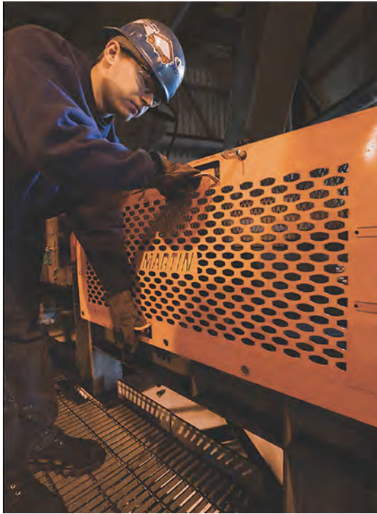
All moving or rotating components should be guarded, regardless of location.
