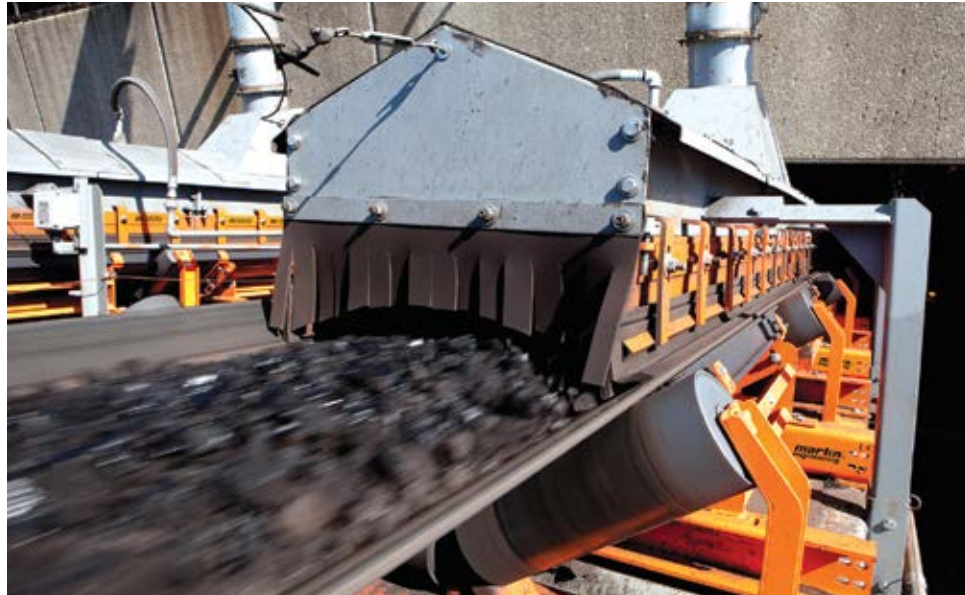
A properly configured conveyor minimizes emissions for improved safety and easier maintenance.
