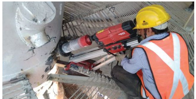
Core drilling during production by a trained technician.
