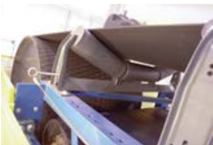
THE PINCH POINT BETWEEN THE BELT AND A CARRYING IDLER IS ONE OPPORTUNITY FOR AN ENTRAPMENT INJURY. © 2020 MARTIN ENGINEERING
